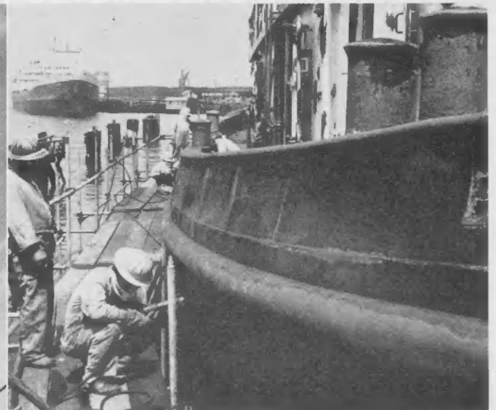
A LIFEBOAT from one of the tugs is swung away effortlessly, a toy for this crane, during the drydocking. Photo at right shows workers cleaning the upper section of the tug's hull as a tanker pulls into the gasoline docks in the background.
